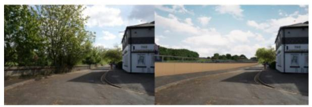
Preston - Riverside: Replacement of the existing concrete wall (left), with a new concrete wall with glass panels on top (right), running on the river side of the road in
